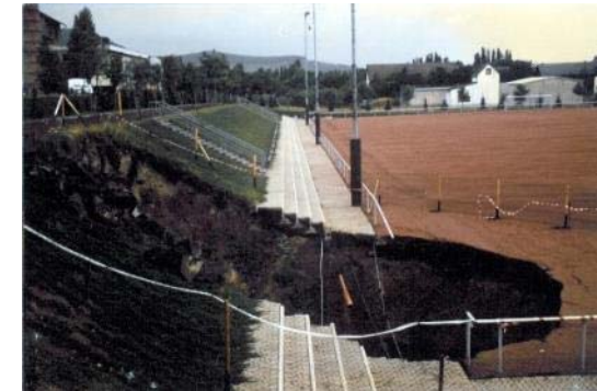
Tagesbruch in Mendig (Foto: LGB)
